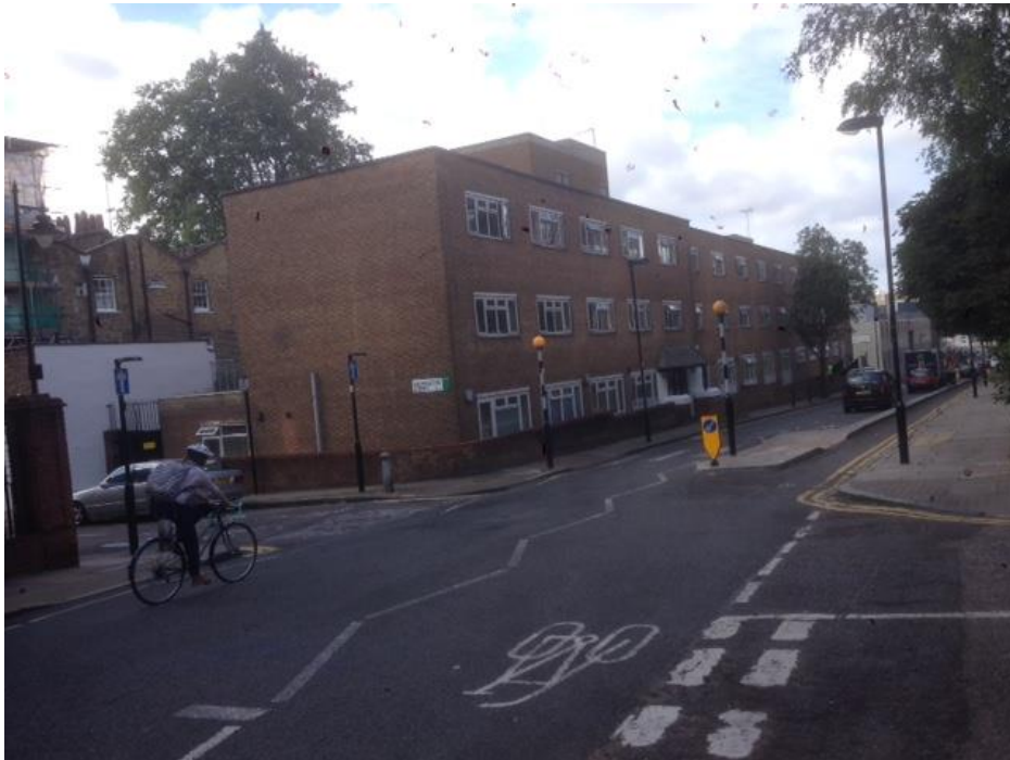
Image 3. 65 Margery Street (looking west)
