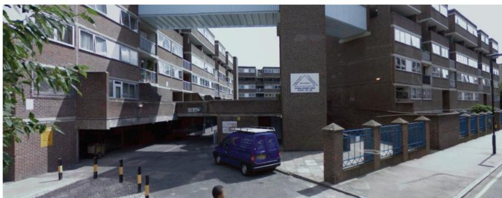
existing Cyrus Street garage entrance
