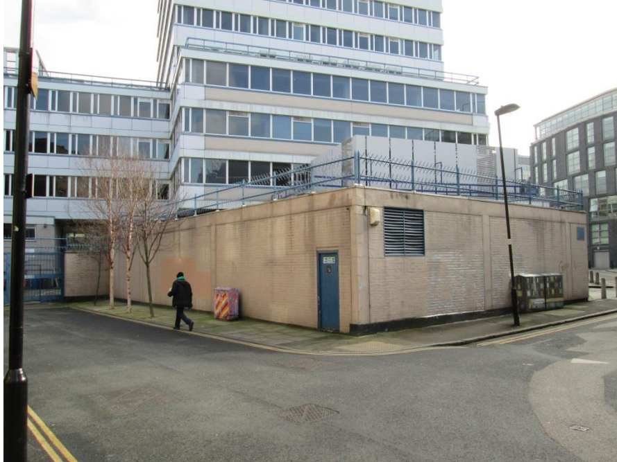
Low rise plant enclosure opposite rear of 1-56 Dufferin Court
