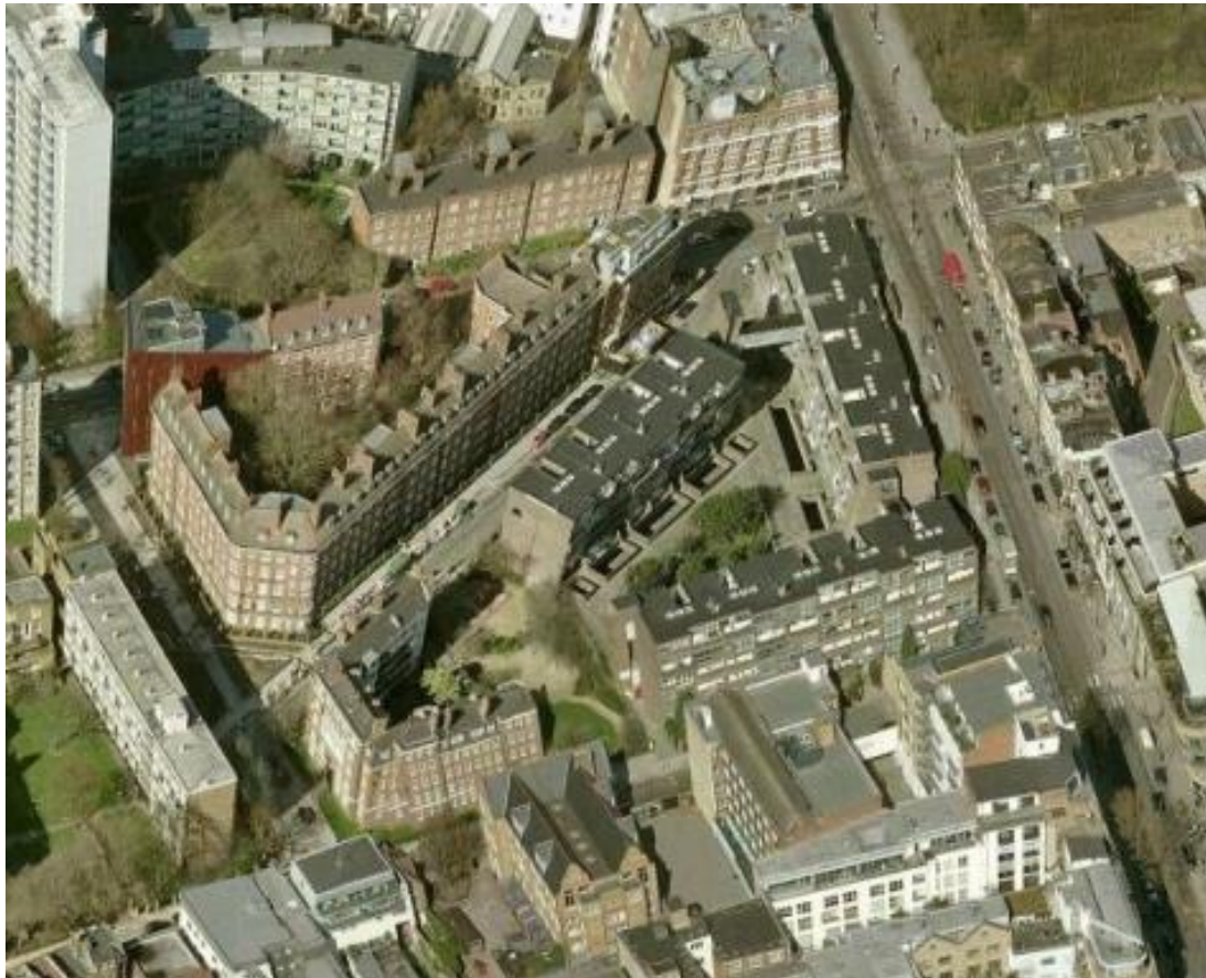
Photograph 1: Aerial View of Site looking north
