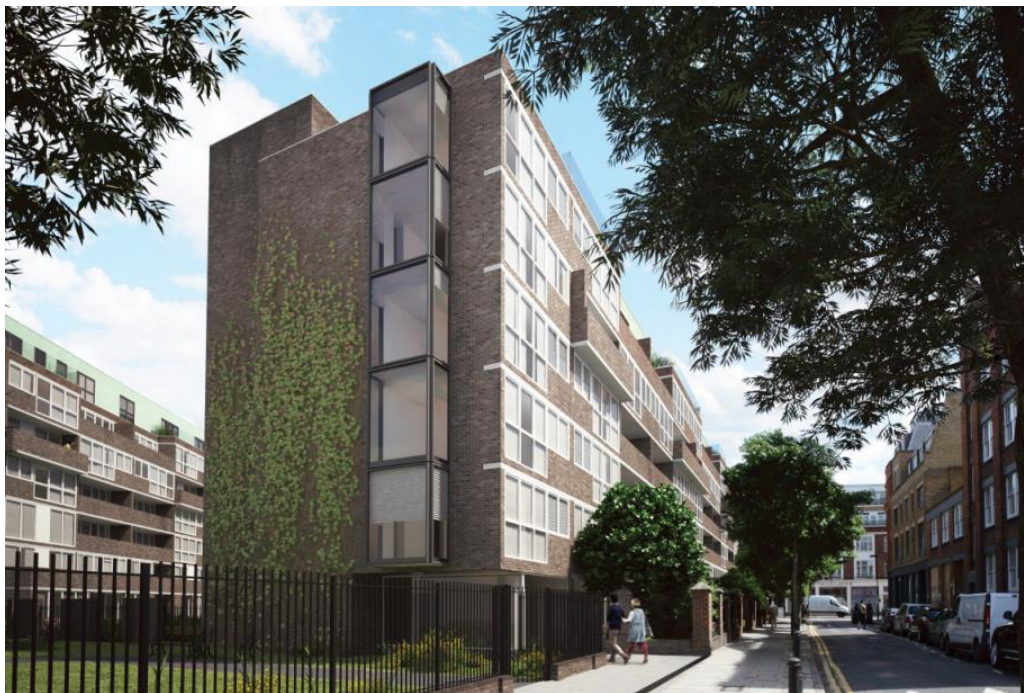
Compton Street Block overlooking Compton Park
